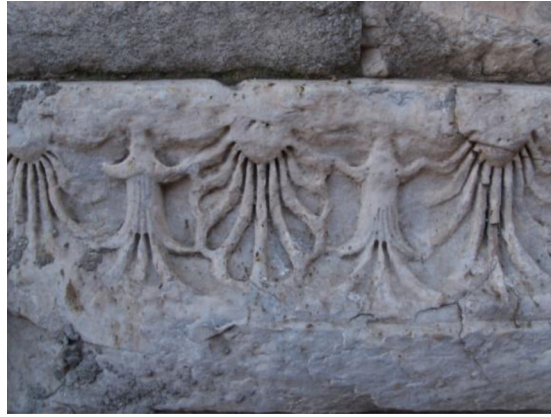
Fig. 7. Deteriorations (external walls).
